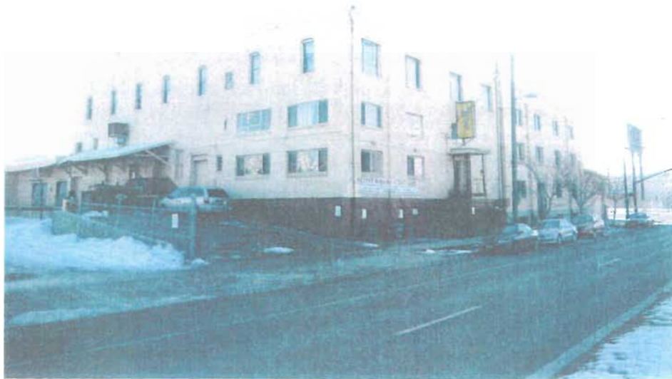
Existing Facility (463 South 400 West)
